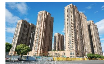
GTR project in Wenzhou, Zhejiang (HK$ 3.7 billion)
