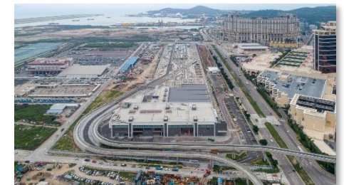
Macau LRT Depot Project (HK$ 1.1 billion)
